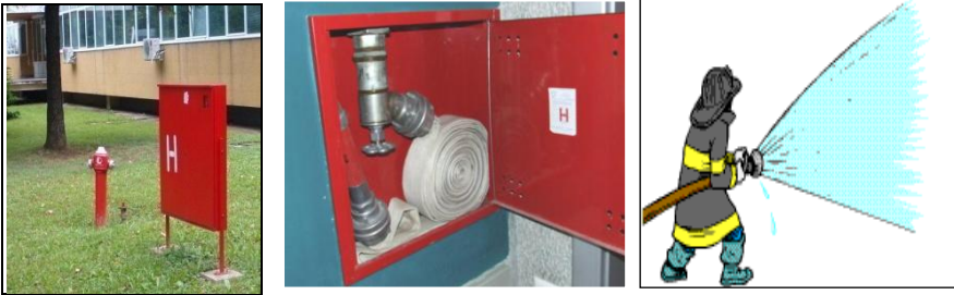
Figure 8. Appearance and method of use of the hydrant
