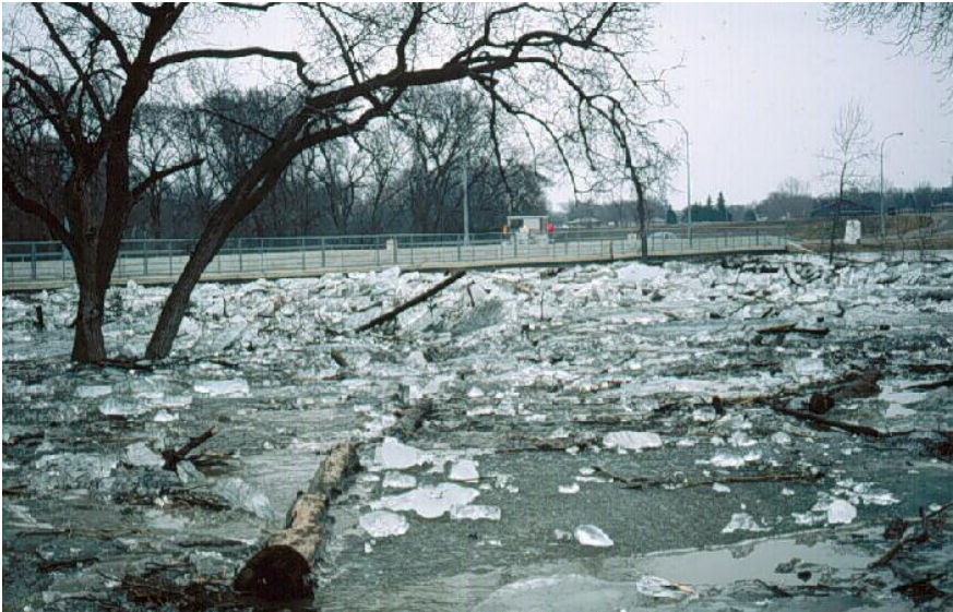
Figure 2. Ice flood - Ice bark creates a plug at the bridge and stopped the flow of the river
