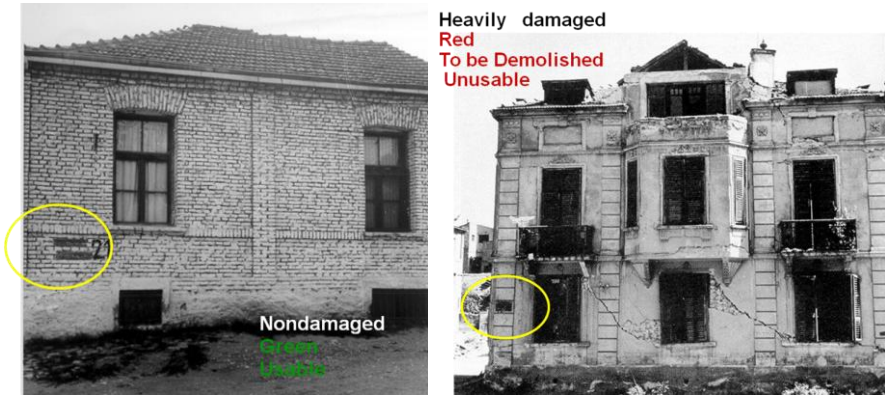
Figure 3. Non-damaged (usable) building (left); heavily damaged (unusable) building (right) [2].
