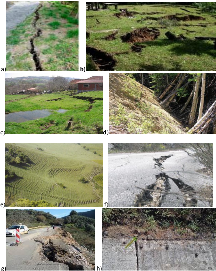
Figure 11. Signs of the landslide outside the settlement: a) cracks, b) scars, c) soil fracture, d) sloping trees e) creeps (slow motion),f) cracks on the road and g) further development of the landslide on the road ,h) starting the support wall of the supporting wall along the dilatation joint
