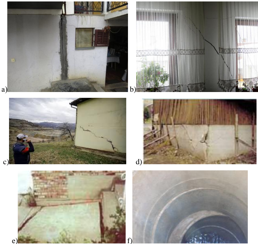
Figure 12. Landlords in the settlement: a), b), c), d) cracks on the walls of buildings, e) cracks on the sidewalk, f) deformed (shifted well)
