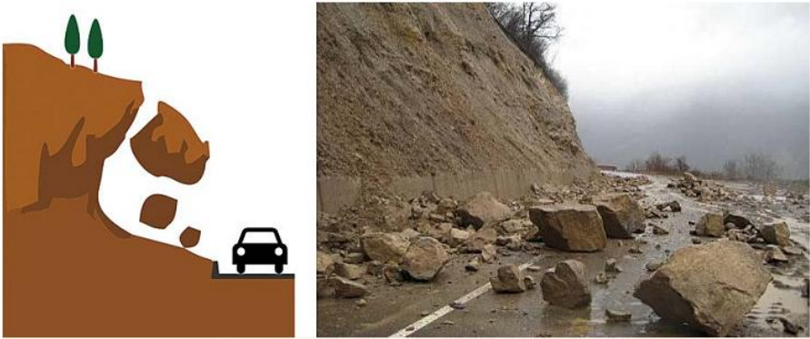
Figure 4. Schematic representation of rockfalls and photographs of field entrances [1]
